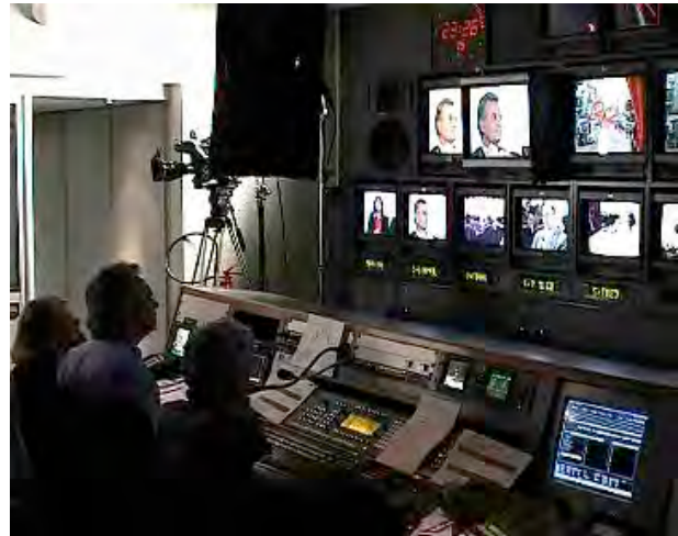
Image 1. The control room
