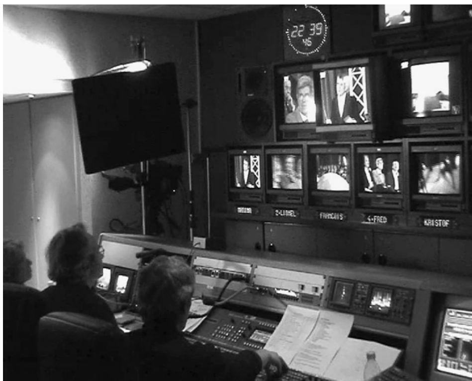
Image 2. Personnel and screens in the control room.
